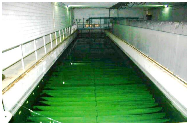
Figure 7 – BAC Filters
