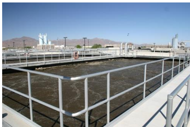
Figure 4 – 1 st Stage Aeration Basin
