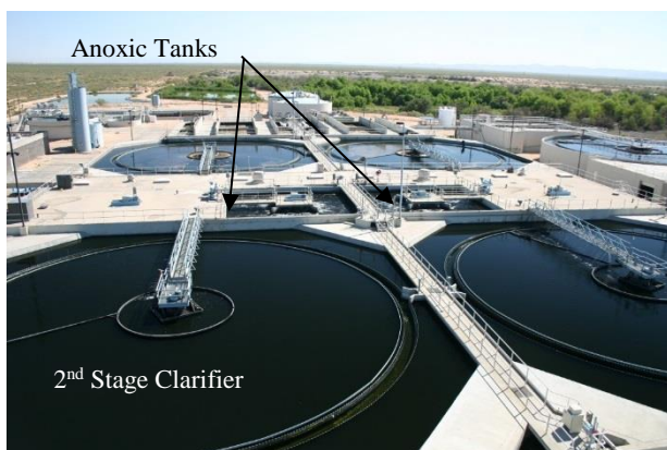
Figure 5 – 2 nd Stage Anoxic Tanks & Clarifiers
